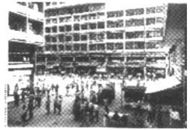
Even on this north facing façade, sun screens are needed. The situation is much worse on west and east facing elevation.
